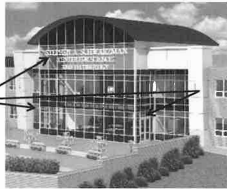
1. Stephen A. Schwarzman Center for Science and Technology (Exterior) September 2020
